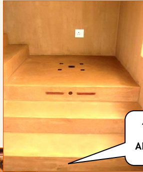
10 - 12 mm Industrial Decorative Coloured Overlay ADCO POLYCRETE 131
