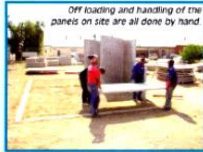
Prefabricated reinforced concrete strips (lintels) forms the foundations for the walls.
